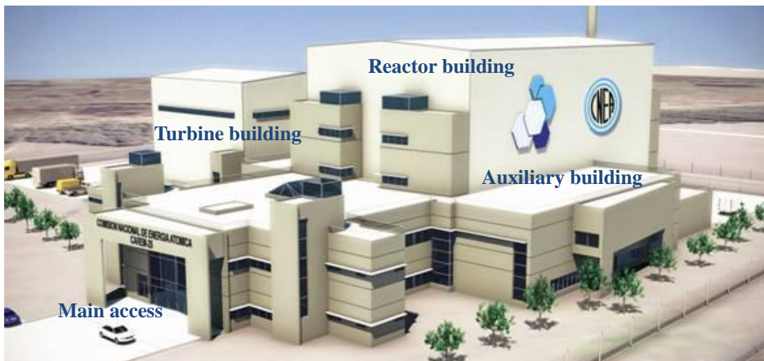
CAREM-25 plant layout (Courtesy of CNEA, with permission)
